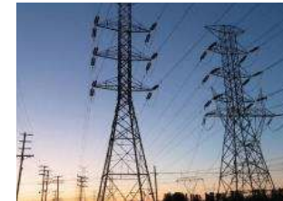
Power distributing Companies
